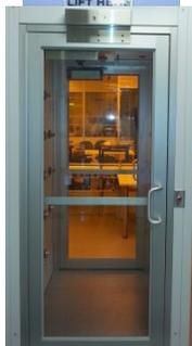
**Air Showers:** For emergency exit, push the **RED** EPO button to disable the interlock of the doors. Under normal condition, the shower will be on automatically when the front door is closed. During the showering, both doors are locked. To prevent contaminates from going through, only ONE door open at a time.
